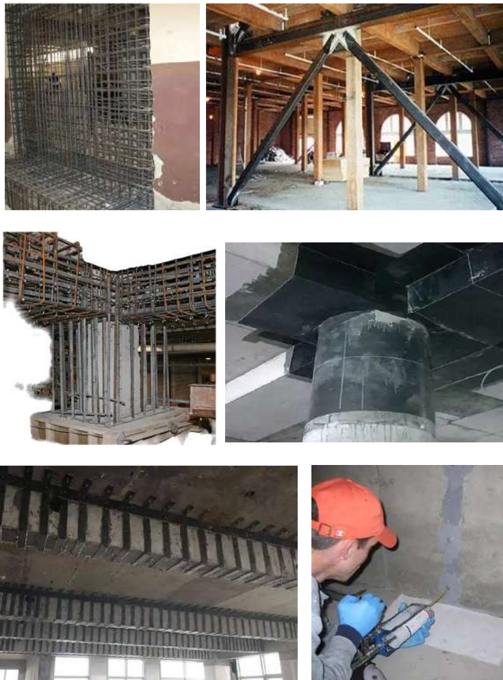
Fig. 10: Retrofitting Solutions (Top Left to Right) Shear Wall, Steel Bracing, Section Enlarging reinforcement, (Middle Left to Right) FRP Reinforced, (Bottom Left to Right) Epoxy Injection Method, External plate Bonding
